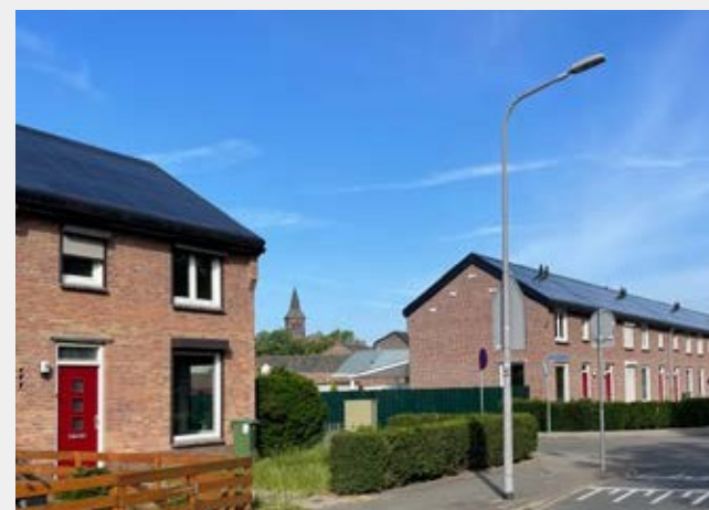
Integrated PV panels on gable roofs
