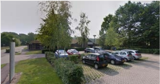
Parking spaces have open paving, allowing rainwater to infiltrate
