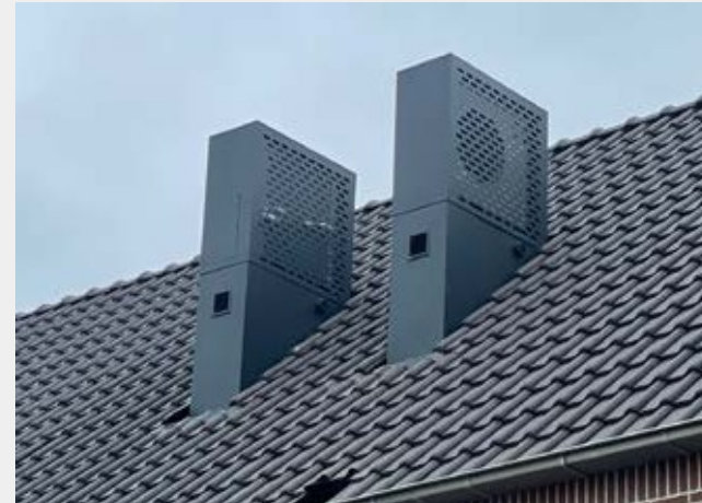
Integrated heat pump as a chimney
