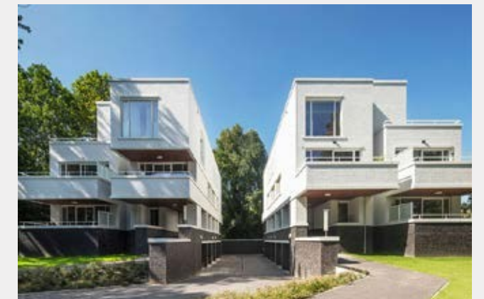
Parklaan Sittard Architect: Humblé Martens & Willems
