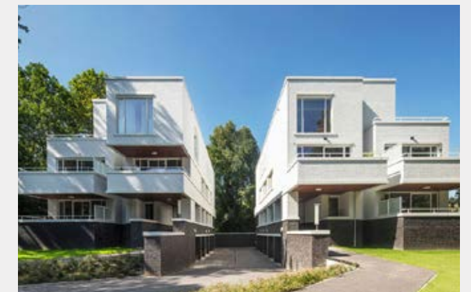
Parklaan Sittard Architect: Humblé Martens & Willems
